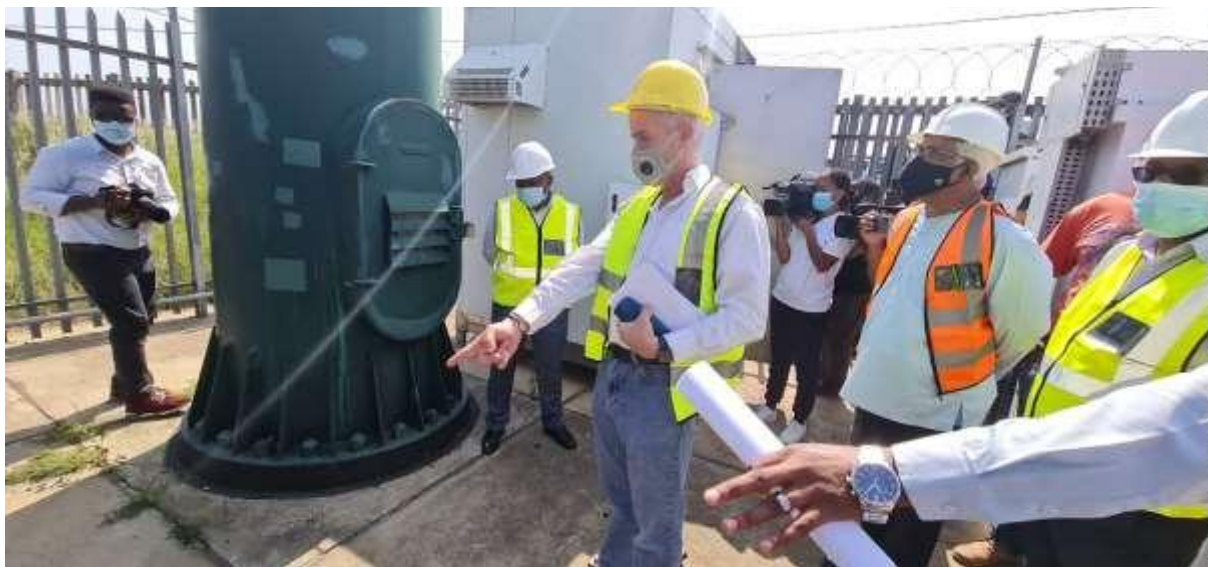
Inspection of a 5G Tower
