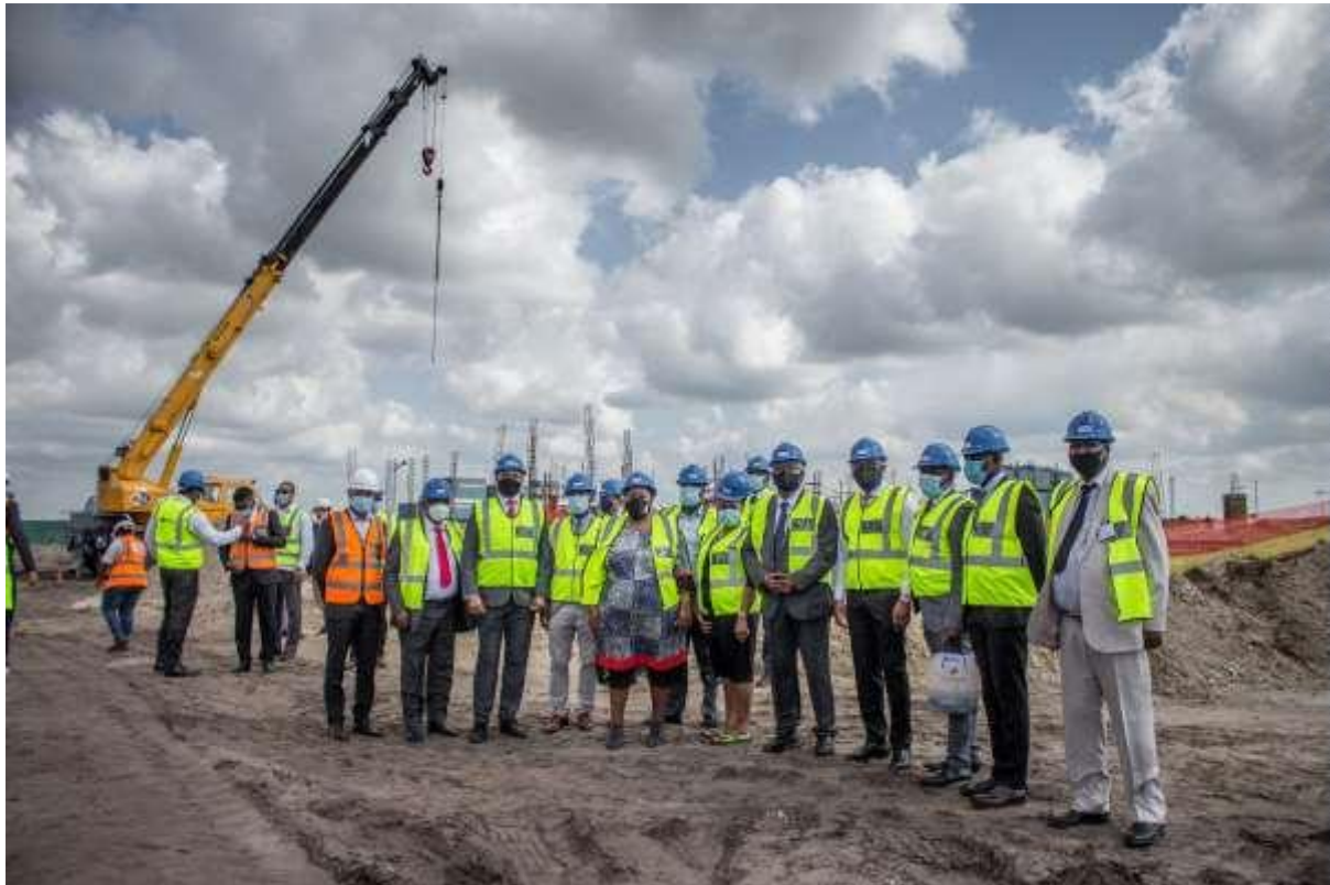
Construction of the first phase of the Nyanza Light Metals titanium dioxide (TiO 2 ) pigment production plant
